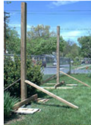
Ensuring the posts remain plumb by bracing them with scrap lumber. David Beaulieu
